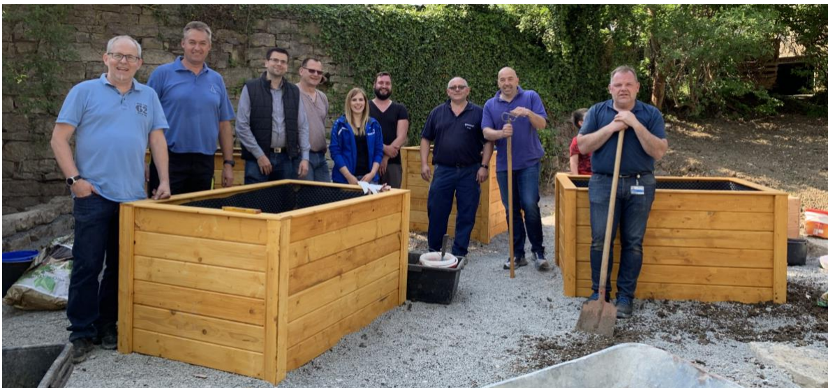
Our engineers with the finished raised beds during the same project in 2019 in Dörzbach.
